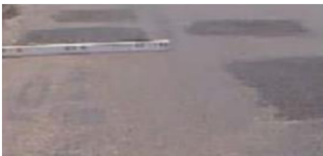
Figure 8. Example of Utility Cut Depression (Direktorat Jendral Bina Marga, 1983)
