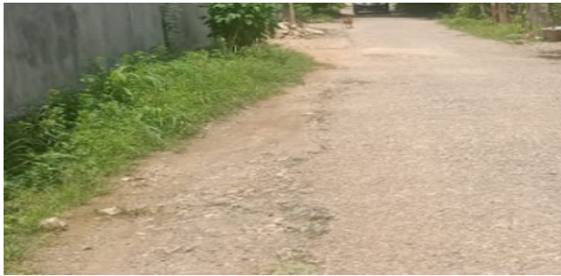
Figure 18. Example of Edge Crack Damage on Location
