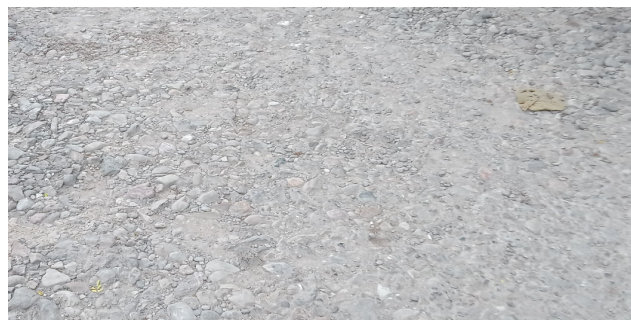
Figure 16. Example of Reveling Damage on Location
