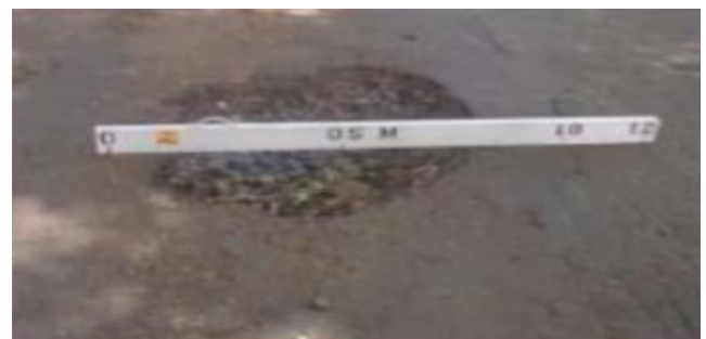
Figure 5. Example of Disintegration (Pothole) (Direktorat Jendral Bina Marga, 1983)
